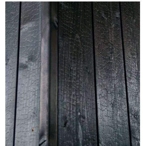
Corner profile: CP3. Painted on site
