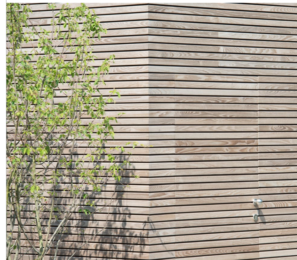
Cut the boards to a 45-degree angle.
